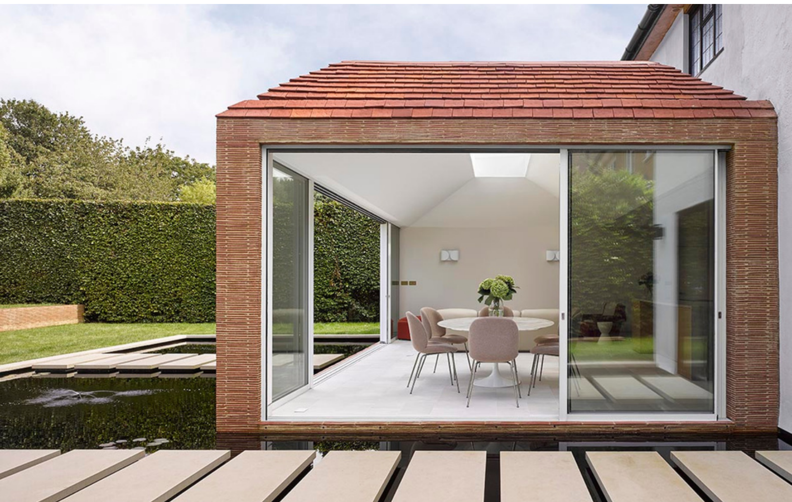
CREASING TILE CLADDING
